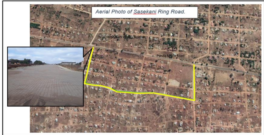
Upgrading of Sasekani Ring Road
