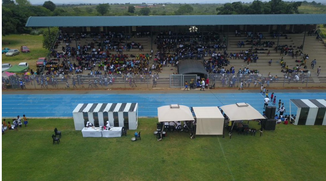
Picture 12 Upgrading of Malamulele Stadium
