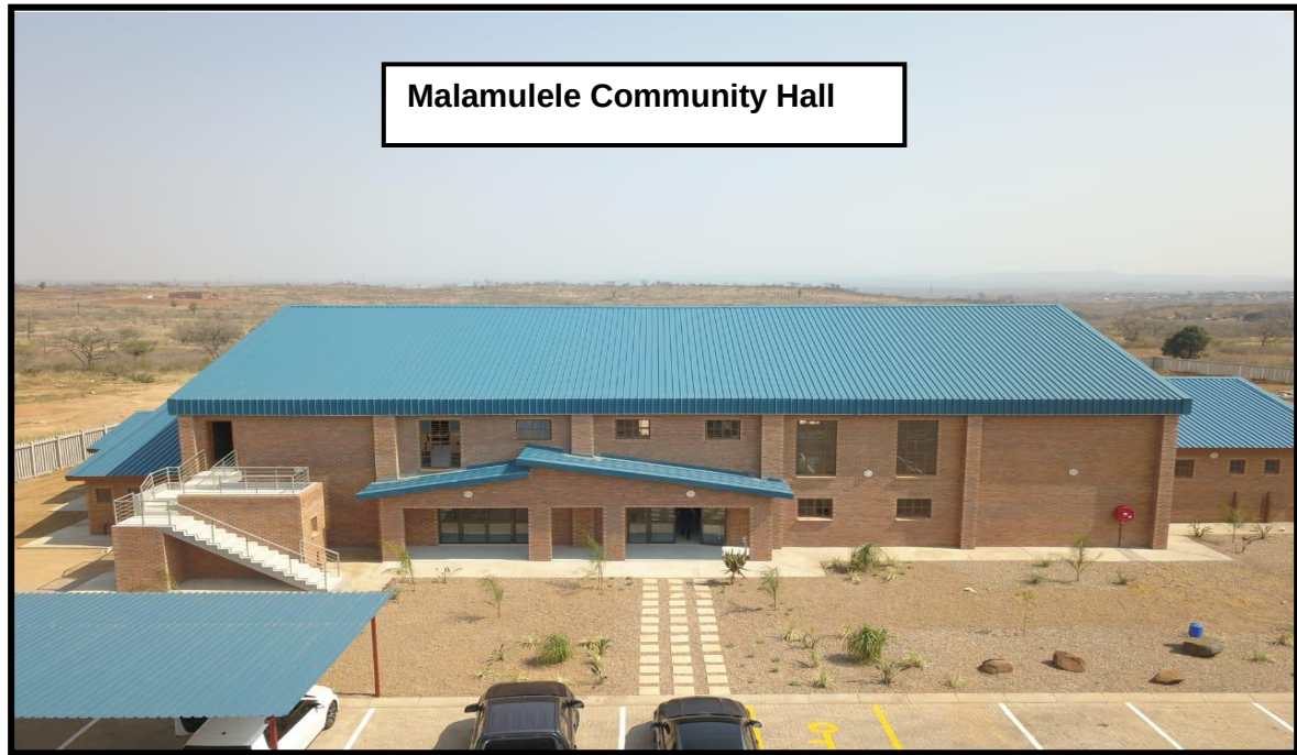
Construction of Malamulele Community Hall
