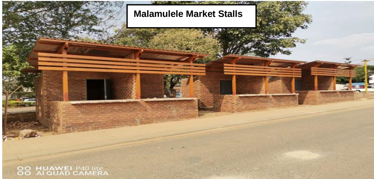
Construction of Malamulele Market Stalls
