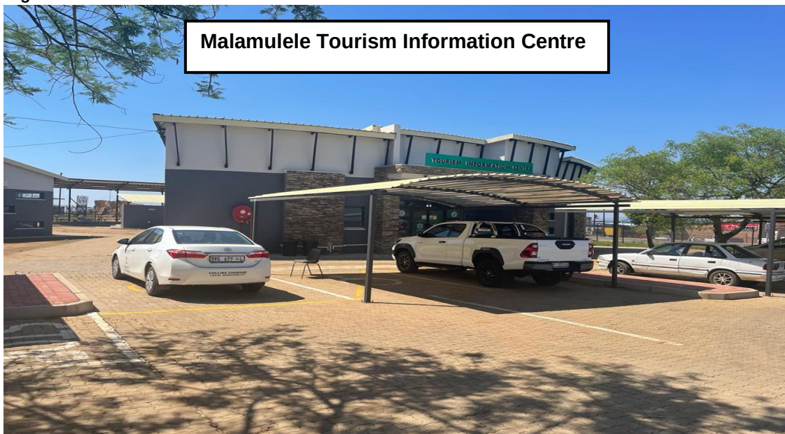
Construction of Malamulele Tourism Information Centre
