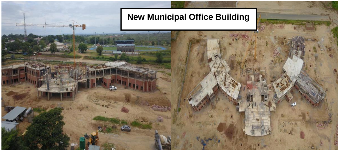
Construction of New Municipal Office Building
