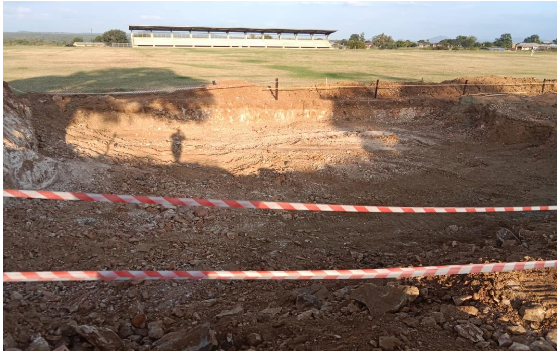
Picture 13 Construction of Davhana Stadium Phase 1
